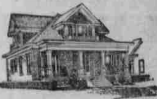
A No. 4-21W IDEAL Boiler and 422 Ft. of 38-in. AMERICAN Radiators, costing the owner $345, were used to heat this cottage. At this price the goods can be bought of any reputable, competent fitter. This did not include cost of labor, pipe, valves, freight, etc., which vary according to climatic and other conditions.
