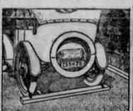
The Use of the Starting Crank and Self-Adjusting Stop Block Makes Hand-Propelling Easy.
