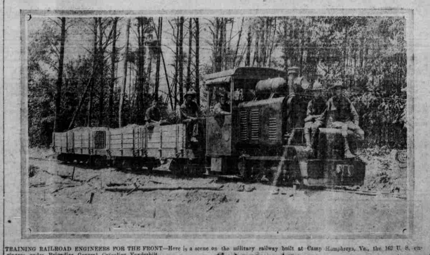
TRAINING RAILROAD ENGINEERS FOR THE FRONT—Here is a scene on the military railway built at Camp Humphreys, Va., the 163 U. S. engineers under Brigadier General Cornelius Vanderbilt.
