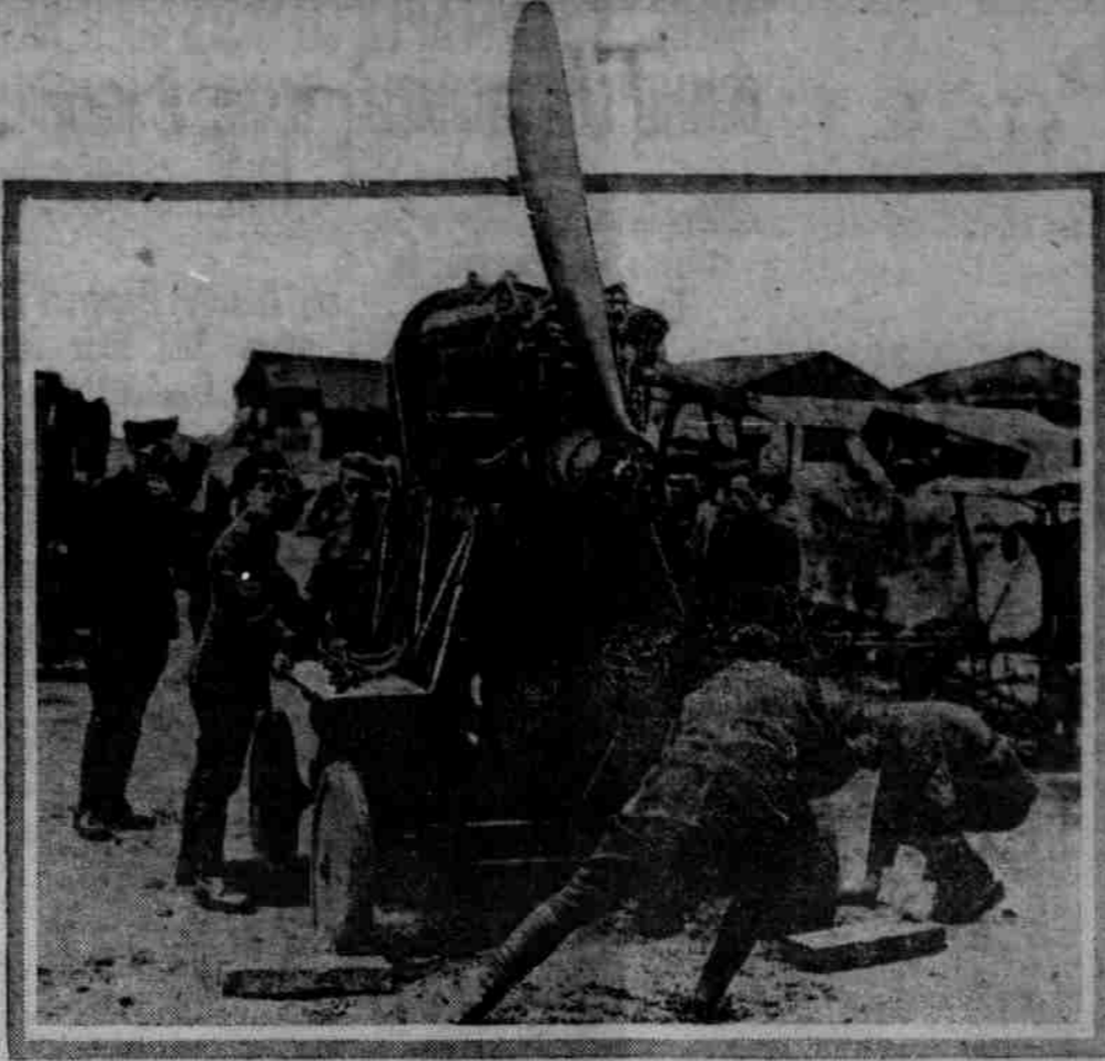
AEROPLANE SALVAGE WORK IN FRANCE —The hospital for damaged airplanes in France is a busy place. This British official photo taken on the British western front in France shows an engine salvaged from a damaged plane being tested.
