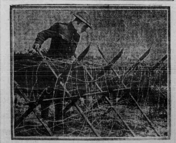
WIRE DEFENSES PLAY A RIG PART-A farmillable wire entanglement which is easily placed anywhere. The frame is of steel bars riveted together and sharply pointed. British official photograph (c) Underwood & Underwood
