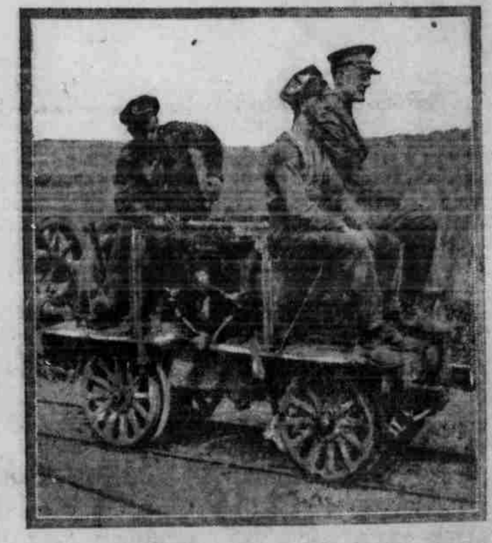
CANADIAN GENIUSES MAKE MECHANICAL BUG--The Canadian official photograph shows the Mechanical Bug, a locomotive made by Canadian corps tramway officers with the help of a corporal. The engine is from a motorcycle, the flue from a once famous sugar refinery and the belt from a mine head now smashed by artillery power.
