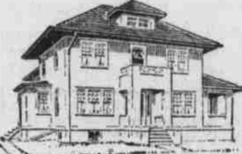
A No. 4-25-9 IDEAL Boiler and 320 ft. of 38-in. AMERICAN Radiators, costing the owner $265, were used to heat this cottage. At this price the goods can be bought of any reputable, competent fitter. This does not include cost of labor, pipe, valves, freight, etc., which vary according to climatic and other conditions.
