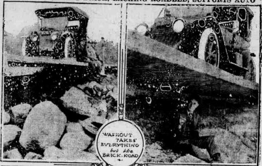
As the result of a spring freshet in Killbuck creek, some sixty square yards of brick paving are doing duty near Wooster, O., undisturbed by the fact that the roadbed beneath is missing.
