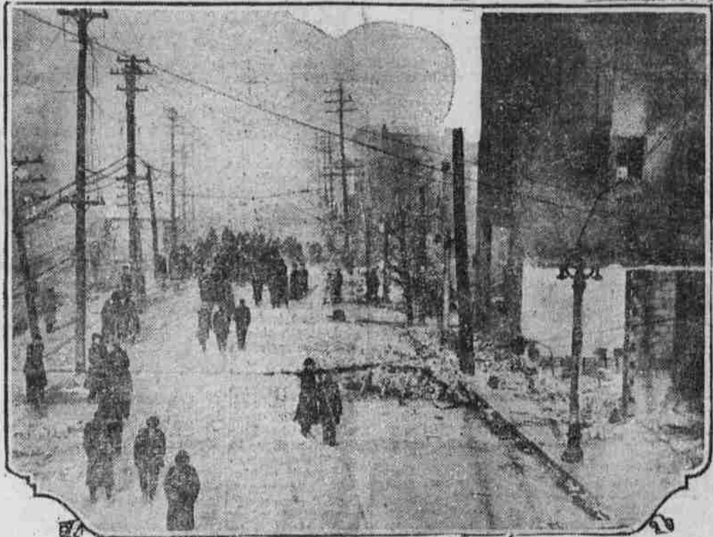
Looking west from bridge on Wilson street, East Youngstown, as strike riot was dying down.
