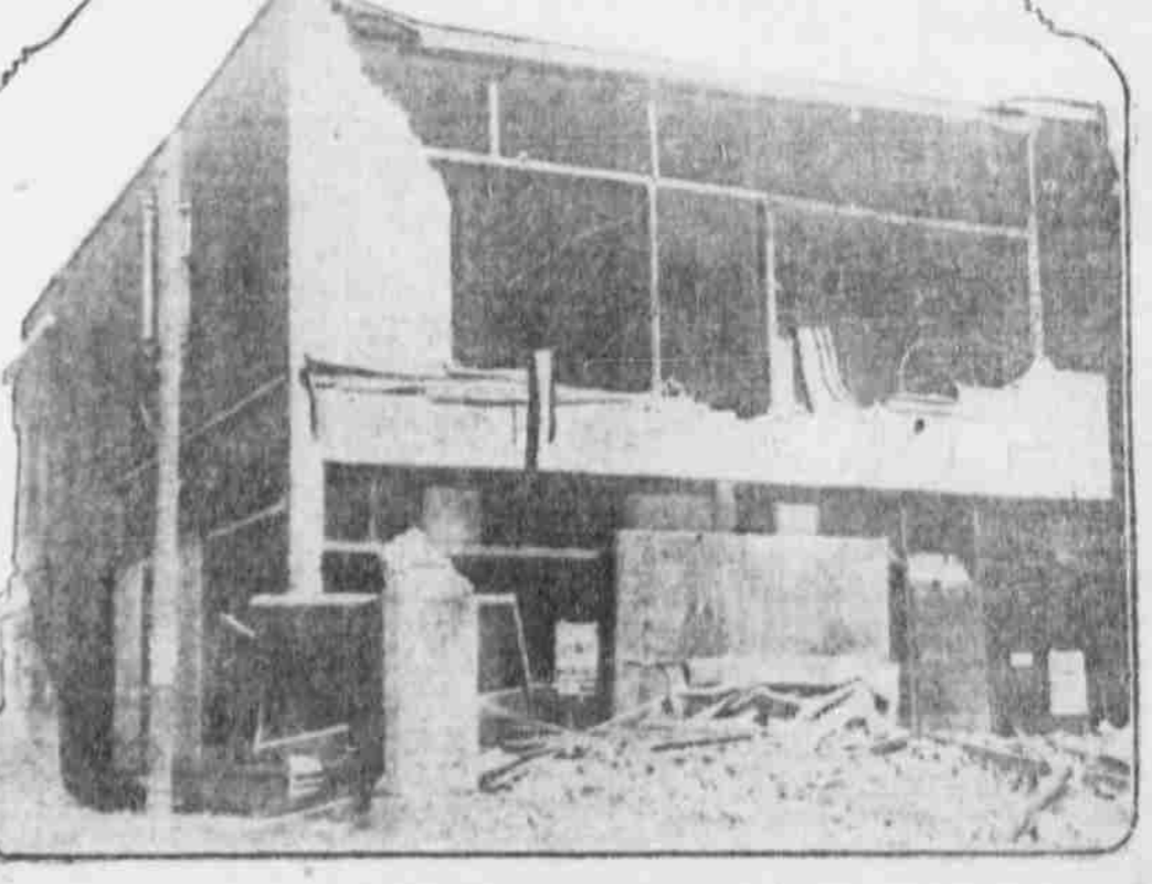
Telephone and telegraph office in El Centro, Cal., after quake. Severe damage amounting to half a million dollars and some loss of life are the results of the earthquake which rocked the Imperial Valley section of southern California. Irrigation works on 400,000 acres of land were endangered and some were destroyed. The severest shocks were felt in El Centro.
