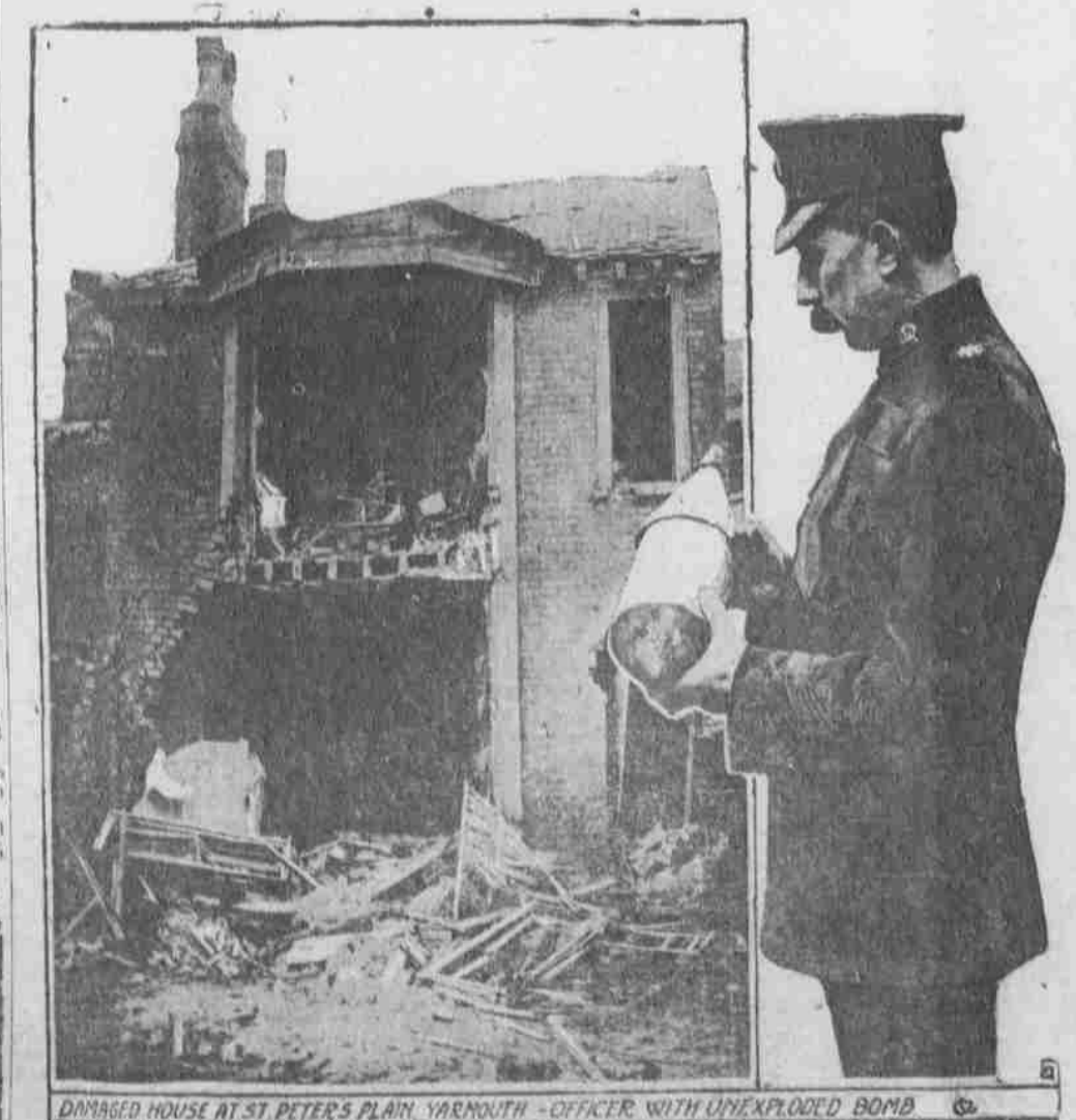
DAMAGED HOUSE AT ST. PETER'S PLAIN, YARMOUTH—OFFICER WITH UNEXPLODED BOMB
