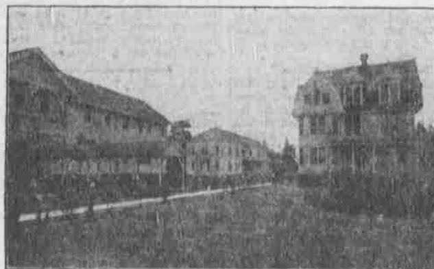
VIEW OF PORTION OF BUILDINGS, COTTAGE FARM, OREGON STATE HOSPITAL, SALEM.
