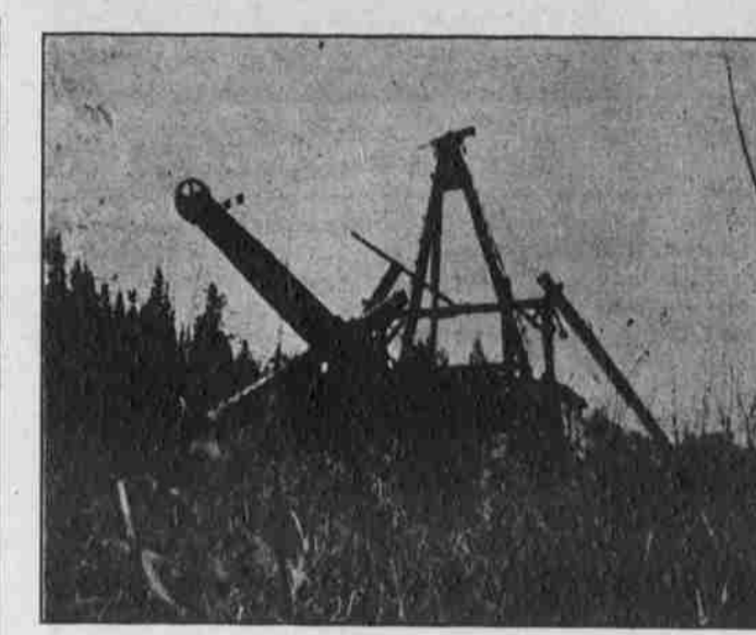
Giant Dredge in Action.
