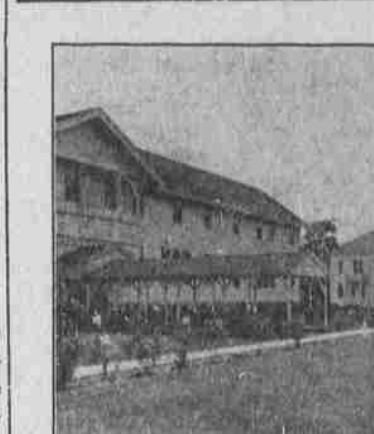
View of Portion of Buildings, Cottage Farm, Oregon State Hospital, Salem.
