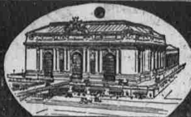
The New Grand Central Terminal New York City
