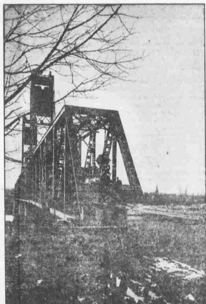
First Train Emerging From East End of the New Bridge.
