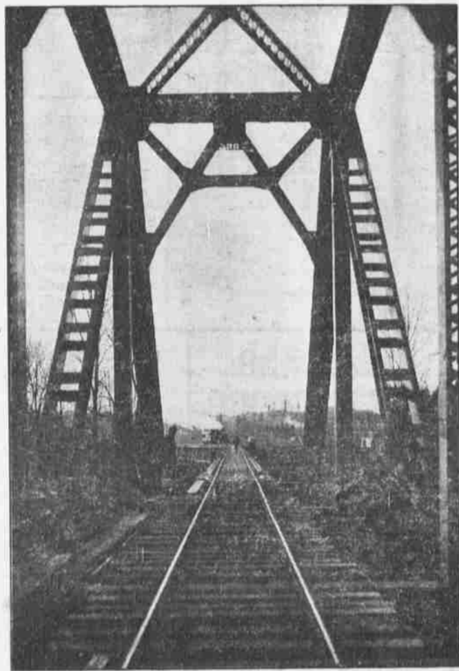
First Train Approaching the West End of New Bridge.
