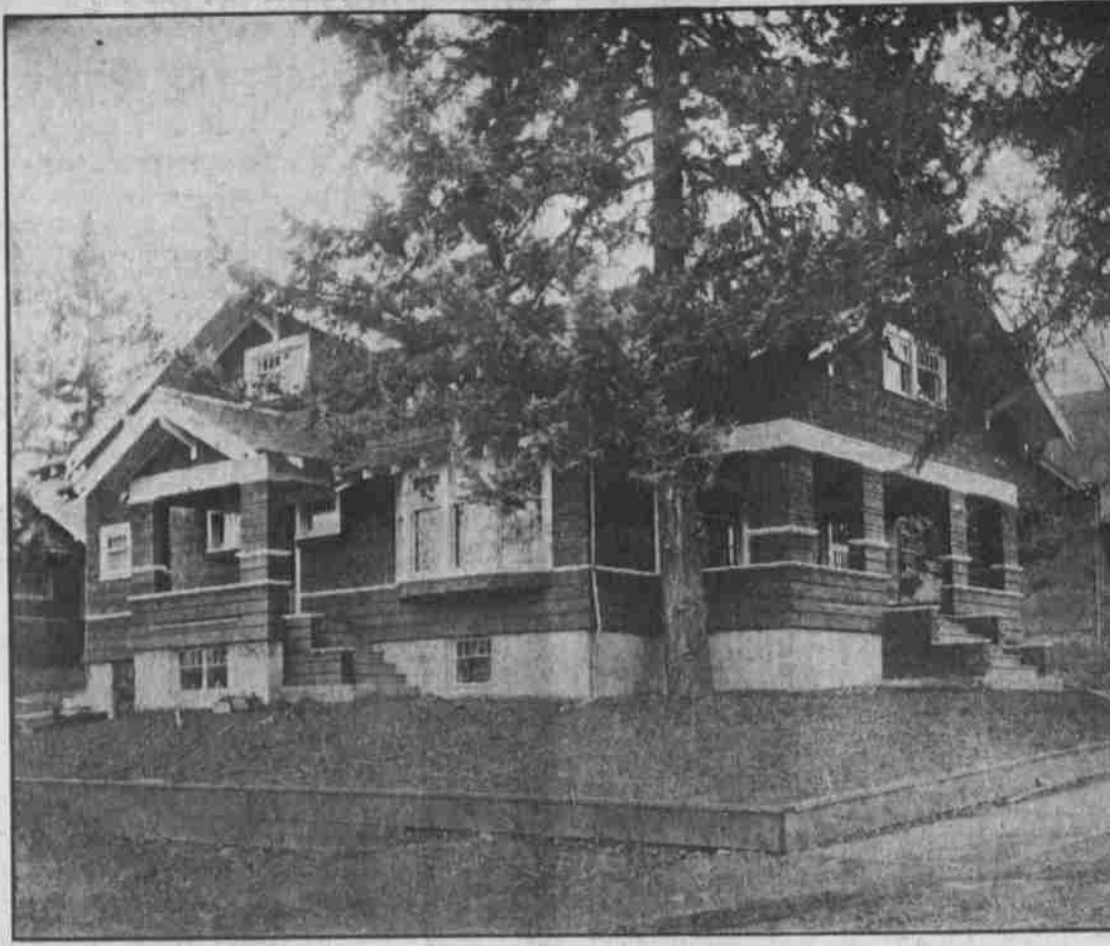
One of the oldest and most reliable contracting firms in Salem is E. Joseph & Sons. These gentlemen not only build houses, but do the architectural work and all designing. Many of the most beautiful houses in Salem have been designed and built by them. The above picture is a good sample of the work which they do. Francis L. Joseph, one of the junior members of the firm, was the designer of the above residence. The modern ideas of the young gentlemen in the firm, together with the substantial old-school building ideas of their father, insure a combination that is bound to please any one for whom they design or build a house.
