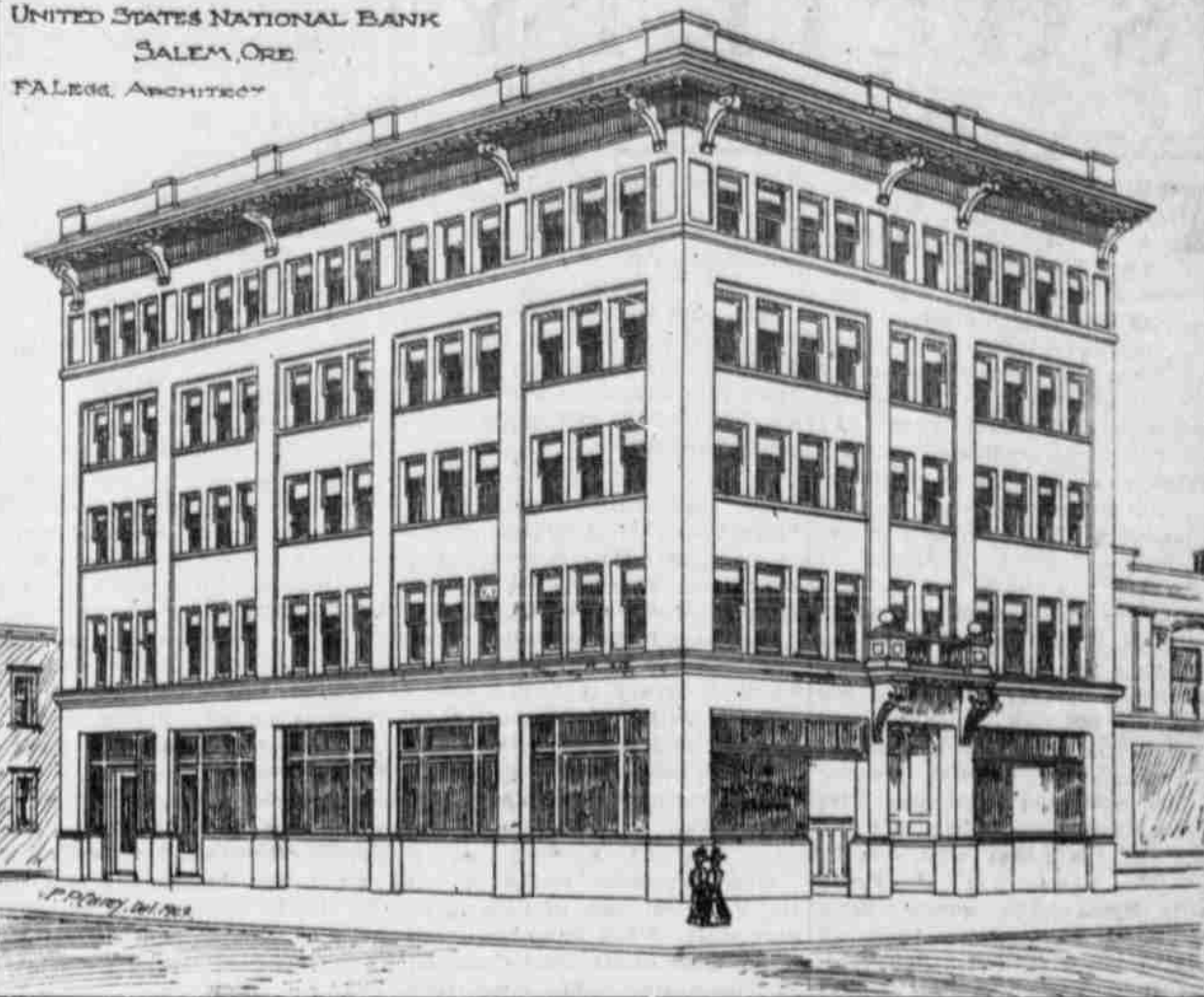
$100,000 FIRE-PROOF STEEL BLOCK BEING ERECTED IN THIS CITY AS A BANK AND OFFICE BUILDING.—See article on Page 2.
