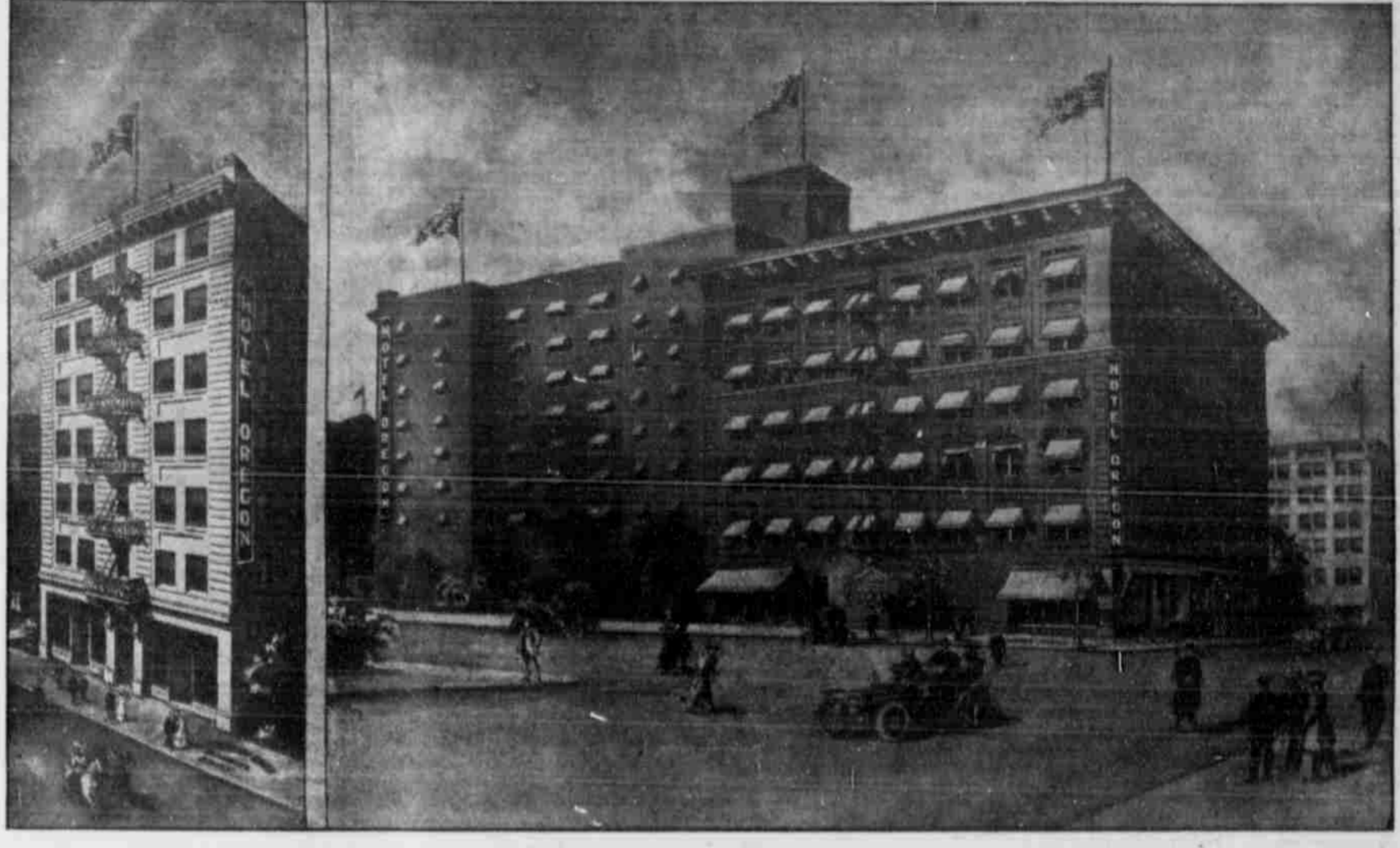
This hotel with its annex just completed and opened to the public has 250 rooms and work will begin with the new year on a seven-story steel frame building on the portion of the lot now covered with a three-story structure. This also will be absolutely fire-proof as is the main part of the hotel and the annex. The hotel is a just source of pride for all true Oregonians, and it enjoys a very large patronage of the best people in the Willamette valley and the whole interior of the state. The Rathskeller grill is without doubt the finest served dining room in the Northwest and has a Hawaiian orchestra and they sing their native songs.
