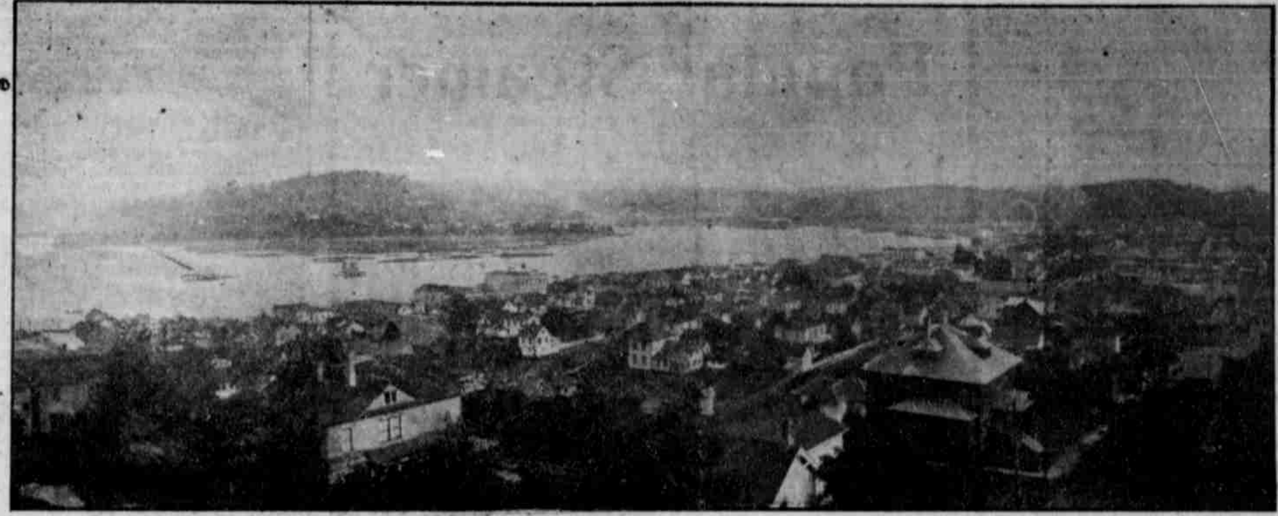
VIEW OF MARSHFIELD, METROPOLIS OF COOS BAY.
