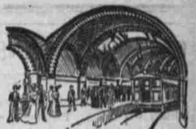
CITY HALL STATION, NEW YORK. Underground Rapid Transit.
