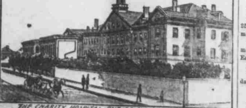
THE CHARITY HOSPITAL, ONE OF THE DANGER SPOTS.
