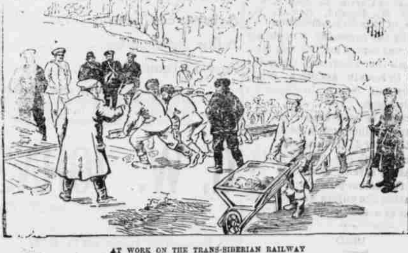
AT WORK ON THE TRANS-SIBERIAN RAILWAY
