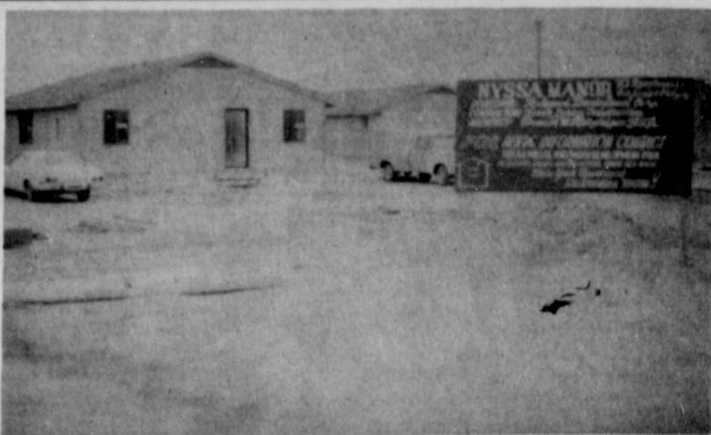
NYSSA MANOR, senior citizen complex for 20 units located in the 500 block on South Fifth Street, is rapidly nearing completion.
