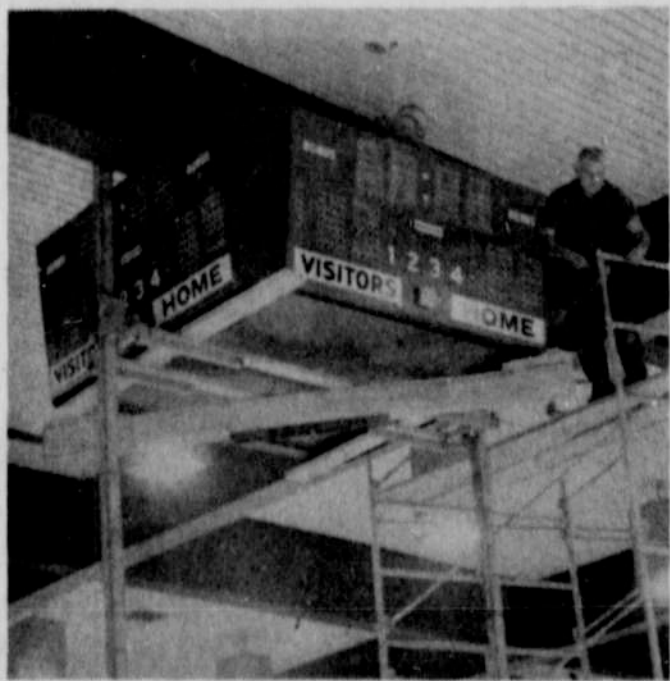
THE NEW SCOREBOARD is being installed securely on overhead beams in the new gym by Merildean Robbins and Lloyd Cannady. It is placed over the center of the basketball floor, and is visible on all four sides.
