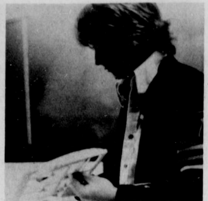
BILL TENSEN, caught in a touchy moment, is seen gluing the spars into the wing of his aircraft.
