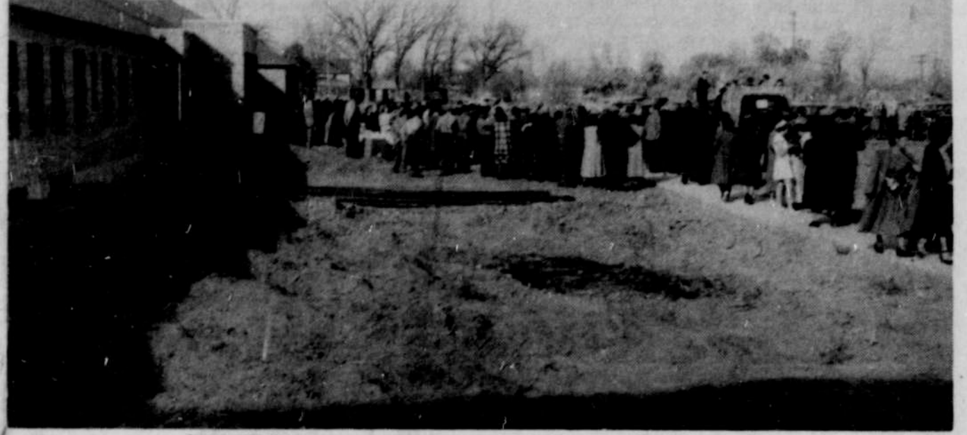
OPENING DAY at Malheur Memorial Hospital September 24, 1950.
