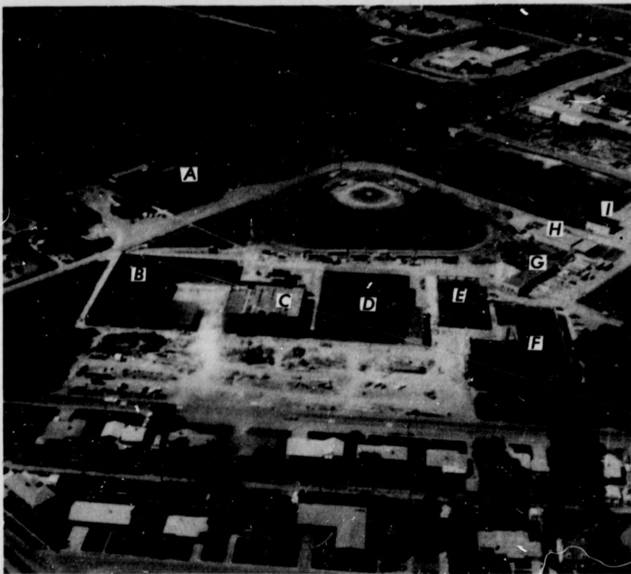
THIS AERIAL PHOTOGRAPH taken by Architect Bob Smith shows the arrangement of the new Nyssa school buildings rapidly nearing completion.
