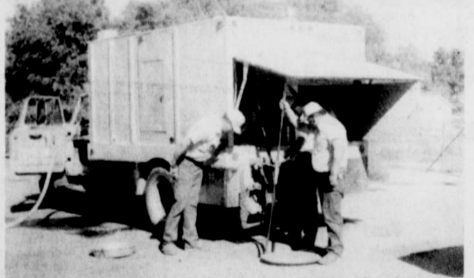
1200 FEET OF SEWER LINE was cleaned of silt earlier this week between the railroad tracks and the Nyssa sewer treatment plant. Shown above is the City of Ontario machine and operator, with Dean Winchester and Steve Marez helping.
