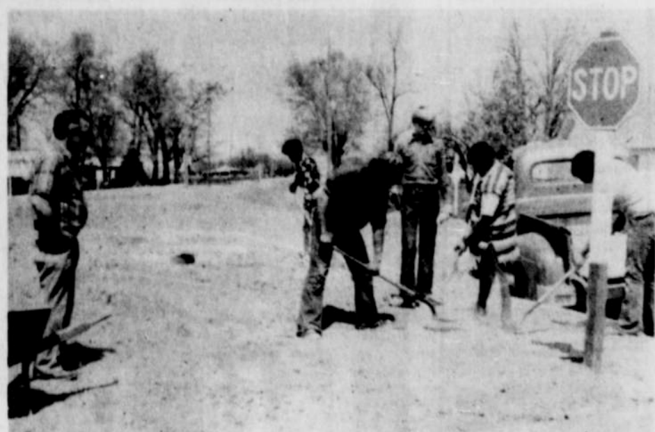
THE BUILDING TRADES CLASS, taught by George Fanning, left, has been busy adding a Bicentennial decoration to the triangle at the north city limits. They have constructed wood lettering with "1776" and
