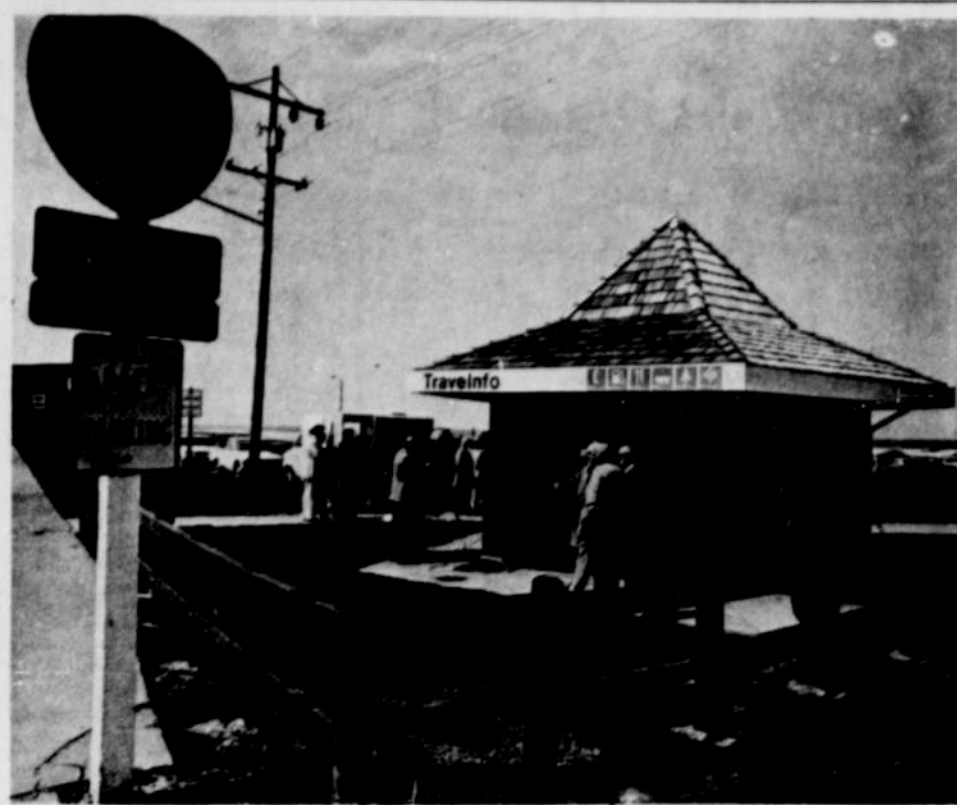
DEDICATION OF THE FIRST TRAVEL InfoCentre on the Oregon Coast was held last week at the D River Wayside in Lincoln City. Covered structure is located just off Highway
