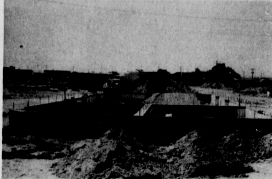
FOUNDATION FOR THE MECHANICAL of the bus garage. building is completed. It is located just south
