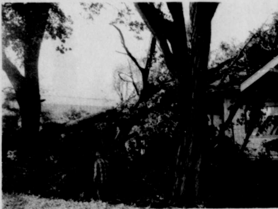
THE L. E. ROBBINS HOME three miles north of Nyssa was damaged by a fallen tree—
