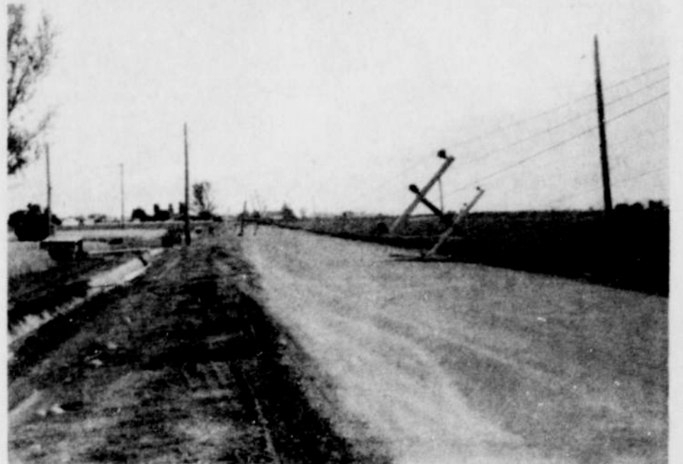
POWER LINES ON ARCADIA BLVD. were felled for a distance of three miles south of Ontario.
