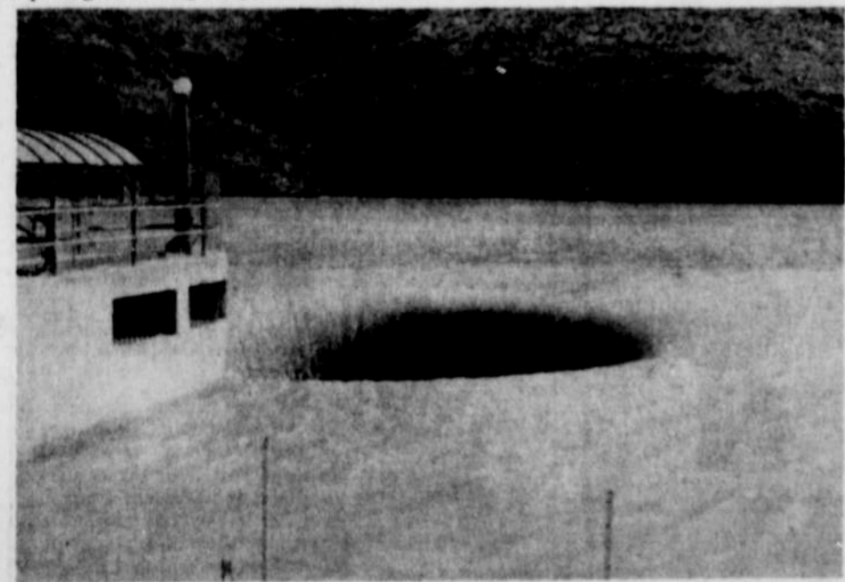
THE GLORY HOLE behind Owyhee Dam is an awsome sight as high water continues to flow over the ring. The high water will
