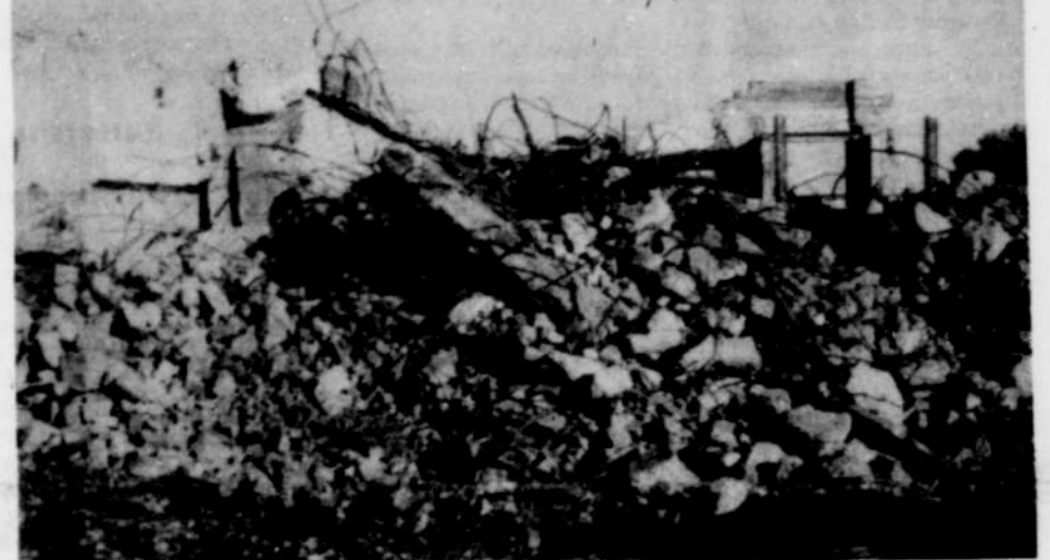
The burned out high school is coming down and being swept up piece by piece. Above the walls are still standing in portions of the destruction while some of the debris has been swept into a junk pile.
