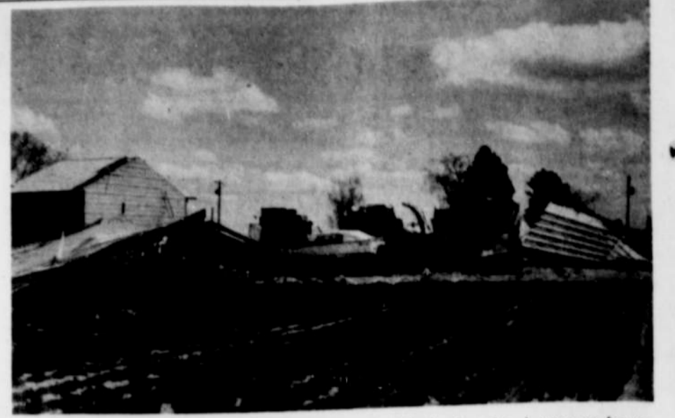
THIS IS WHAT WAS LEFT OF A LARGE 3-bay machine shop on the Robert Munn farm in Sunset Valley, after it was hit by a twister Tuesday, April 23 about 5 p.m. The building housed three large combines, a camper, a boat and miscellaneous items, most of which were damaged. The twister
