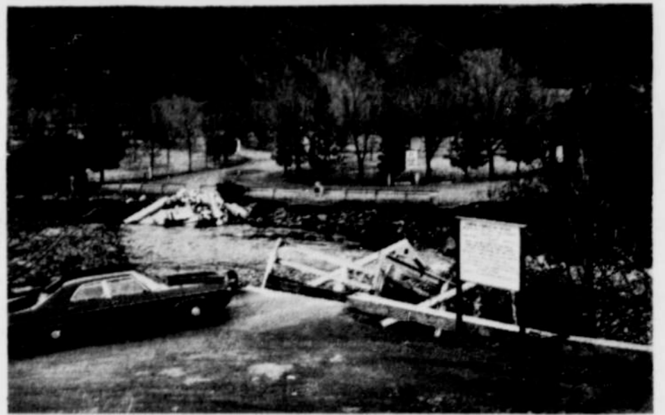
ACCESS BRIDGE (center) to Idaho Power Company's McCormick Park near Brownlee Dam collapsed into Wildhorse Creek when the stream, swollen by heavy rains and snow melt, cut away both its banks. On opposite side of creek are ruins of the park's restrooms, also damaged by the high water.
