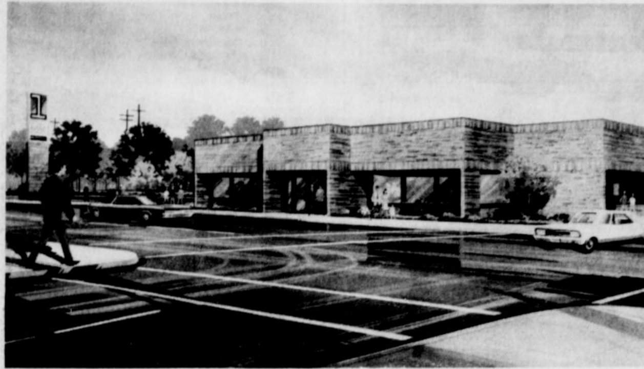
THE NYSSA BRANCH OF FIRST NATIONAL BANK OF Oregon will look like this when this new building is completed during the Fall of 1974. The exterior will be giant brick masonry units with bronzed glass and a roof constructed of built-up frame trusses. Plans call for extensive landscaping at the site with 21 off-street parking stalls.
