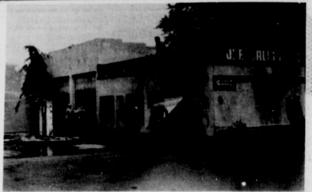
NYSSA VOLUNTEER FIREMEN battle a blaze that erupted in the old service station behind Ray's Food Fair last Friday afternoon. The building has been un-
