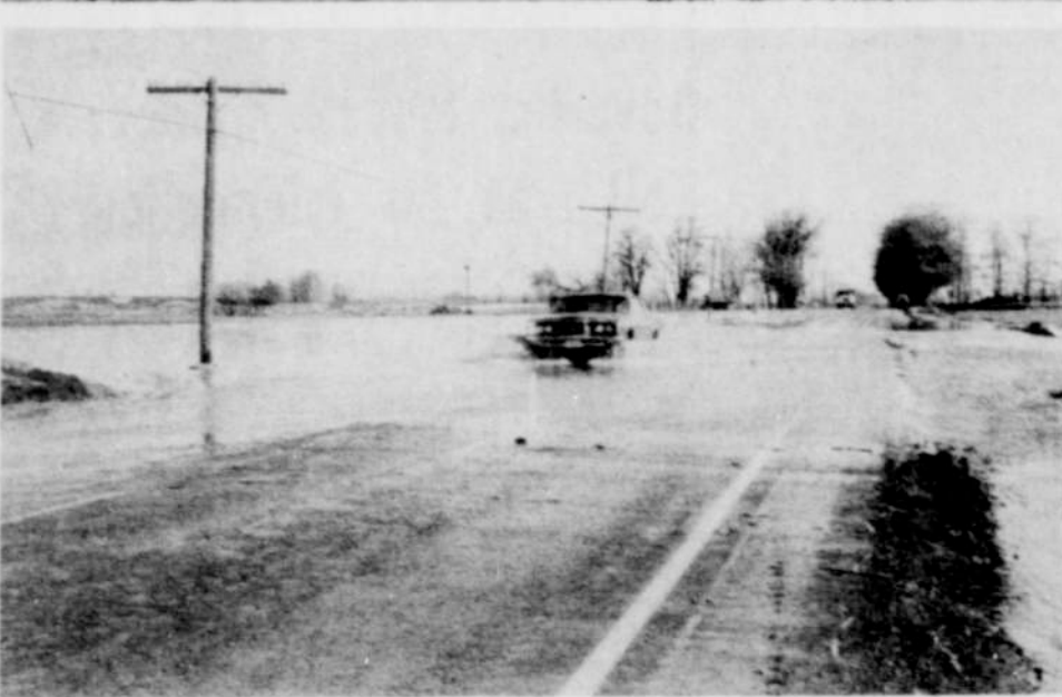
THE OWYHEE DITCH BROKE five miles north of Nyssa early Friday morning, flooding fields and running over Highway 201 near Imperial Avenue.
