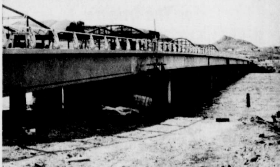
THE NEW BRIDGE AT ADRIAN is rapidly nearing completion, with traffic expected across the bridge by April 23 according to Scott Hanson, project engineer for Willamette-Western Corporation of Portland, who has the construction contract.
