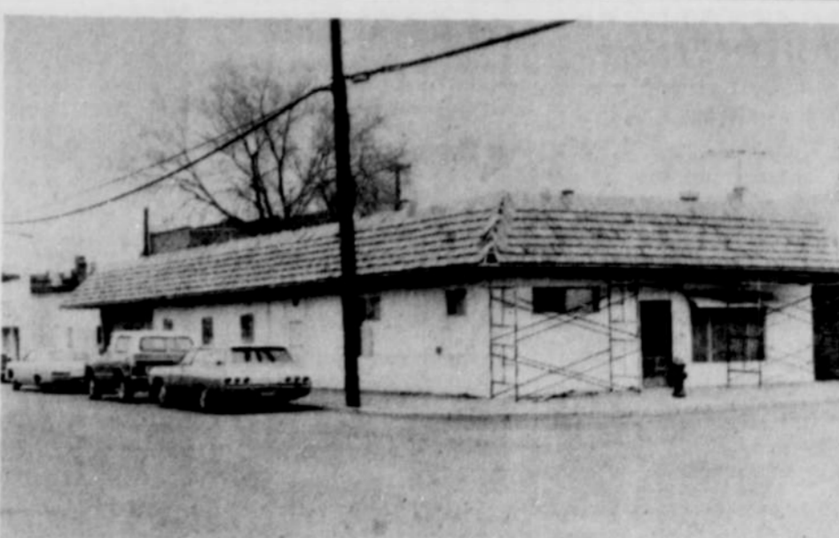
A RUSTIC SHAKE MARQUEE around the newly enlarged clinic of Dr. Charles E. Vanetti at the corner of Second and Good Avenue adds much to the appearance of the building. The new addition is at the far left, and is about to receive a coating of stucco and paint.
