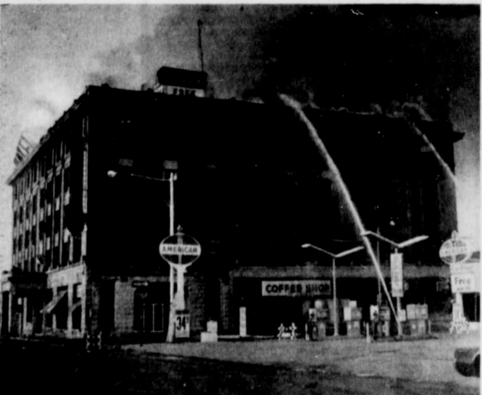
THE HISTORIC WASHINGTON HOTEL in Weiser is only a shell after a fire gutted the old building Friday night. This picture taken Saturday morning shows weary crews still pouring water onto the roof of the building.
