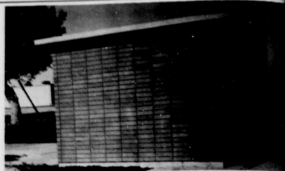
THIS NEW BUILDING on the TVCC campus has been recently built on the west end of the Administration Building. It is the storage facility for flammable, corrosive and toxic chemicals used in college chemistry classes. The compact fireproof interior, measuring 6'x6'x8' provides shelving in an atmosphere which ranges between 40 and 70 degrees. A steel door controls access, and a refrigerator is provided for the most highly volatile and instable of the organic chemicals.
