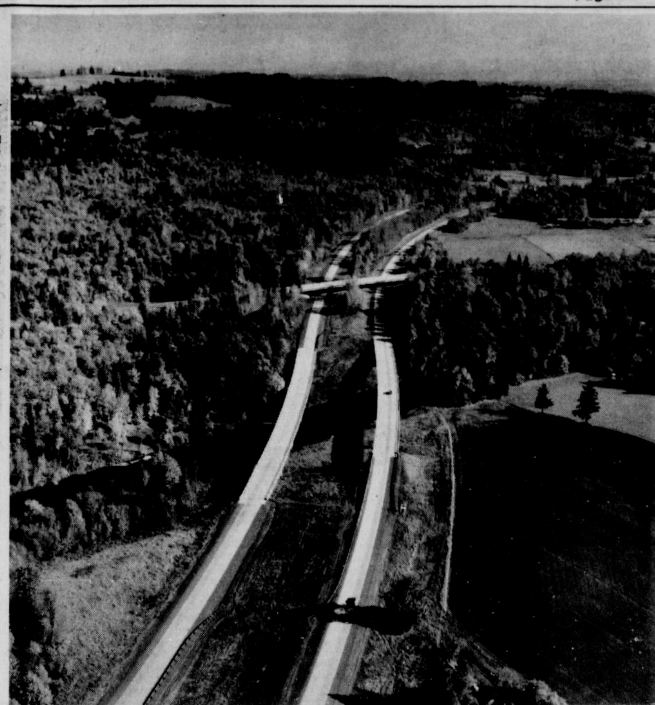
A463-28 - View shows I-205 at its crossing of the Tualatin River. Just beyond, freeway goes under a county road overcrossing structure. (Oregon State Highway Division photo)
