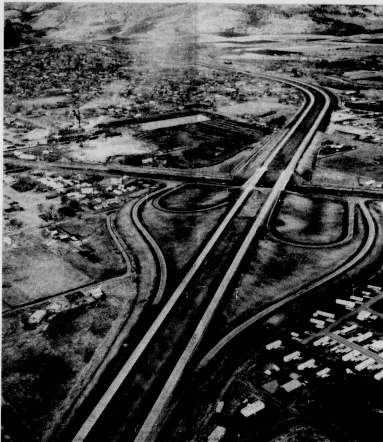
A464-9 -- View is northwesterly, showing I-80N bypass of LaGrande, upper left. In center is the Wallowa Lake Highway Interchange. (Oregon State Highway Division photo)
