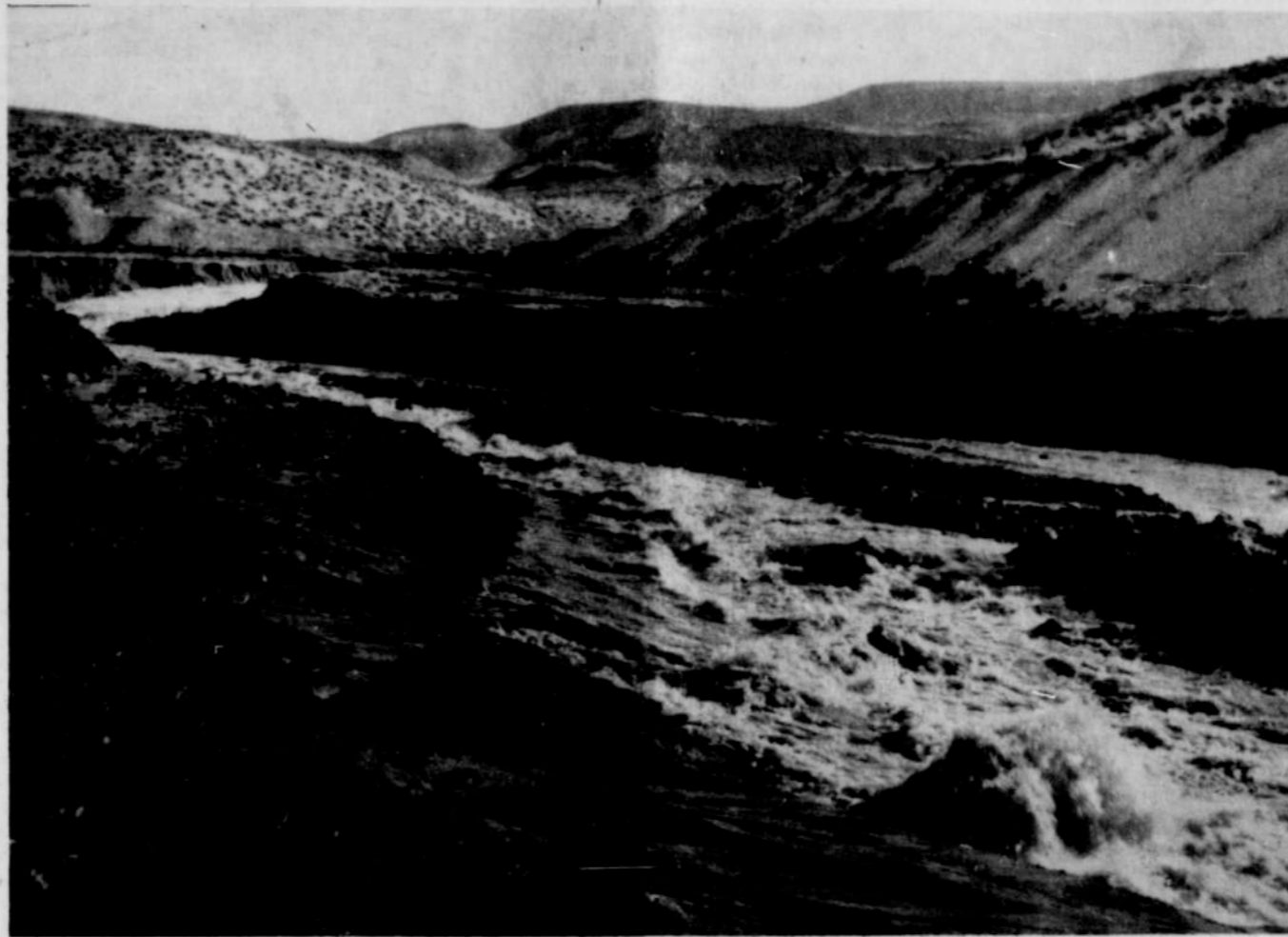
This gully was carved by water from a Vale, Oregon Irrigation district canal which broke near Harper early Tuesday morning. The canal break caused considerable damage before the water could be shut off. The water covered
