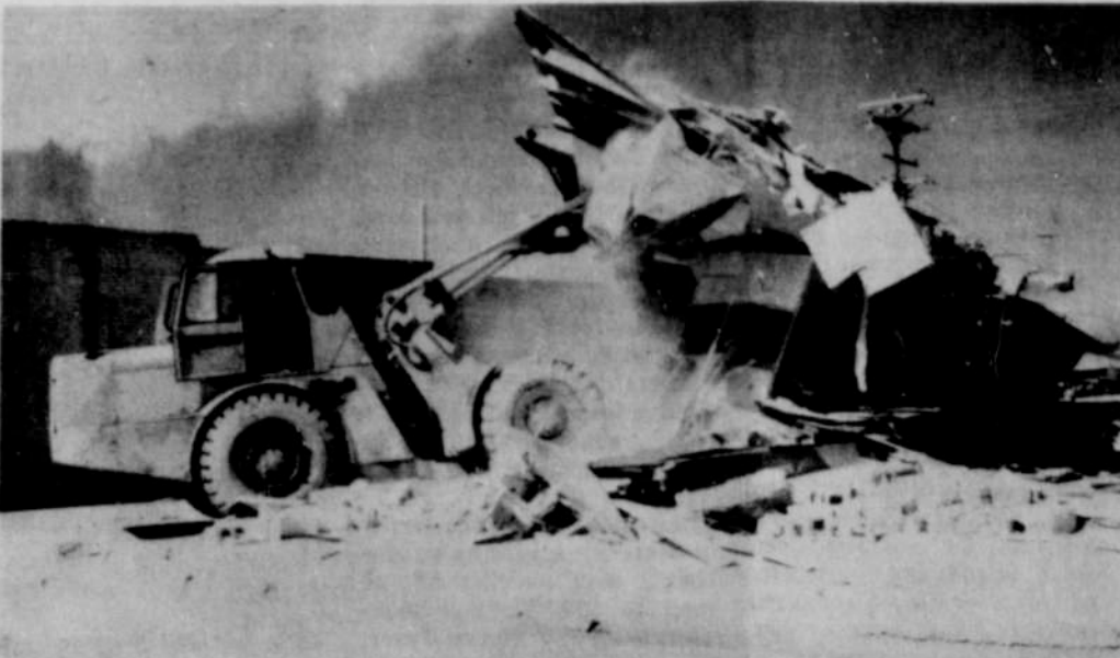
THIS IS THE FINAL PUSH ON THE POLAR Bear building (pictured in the Journal two weeks ago). The scoomobile collapsed the wall and started razing the brick building seen at the left. With use of the machine seen here and three trucks both were down
