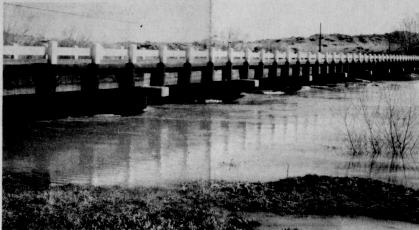
WATER WAS LAPPING AT THE FLOOR OF THE OWYHEE river bridge south of Nyssa Tuesday afternoon. Most of this was from the Owyhee reservoir some 30 miles upstream to the dam. The balance was surface water caused
